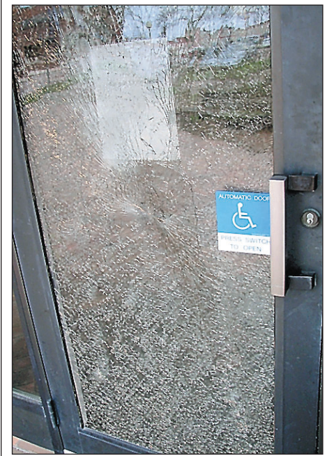
Upon arriving at work the morning of April 11, employees of the Vermillion Public Library found someone had shattered the glass in the building's front door. The entire pane is now a spider web of broken glass and needs to be replaced. A $500 pane has been ordered, but has not arrived yet. The identity of the vandal or vandals is unknown at this time. (Photo by Travis Gulbrandson)
