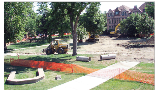
This summer, portions of the University of South Dakota campus have been off-limits to the public as workers replace utility lines. The work is scheduled to be completed this month.
