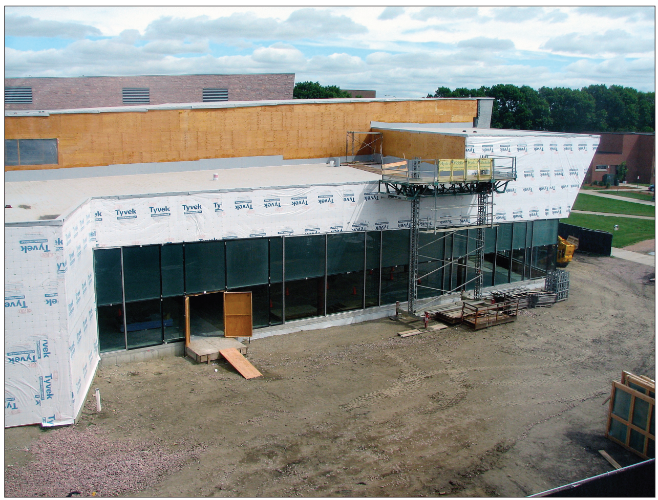
The 31,000 square foot expansion of the Muenster University Center (MUC) began late last fall, with exterior work. Through the spring and summer the project has included placement of additional steel beams, pouring the floors, and work on the exterior enclosure of the new addition. (Photo by Travis Gulbrandson)
