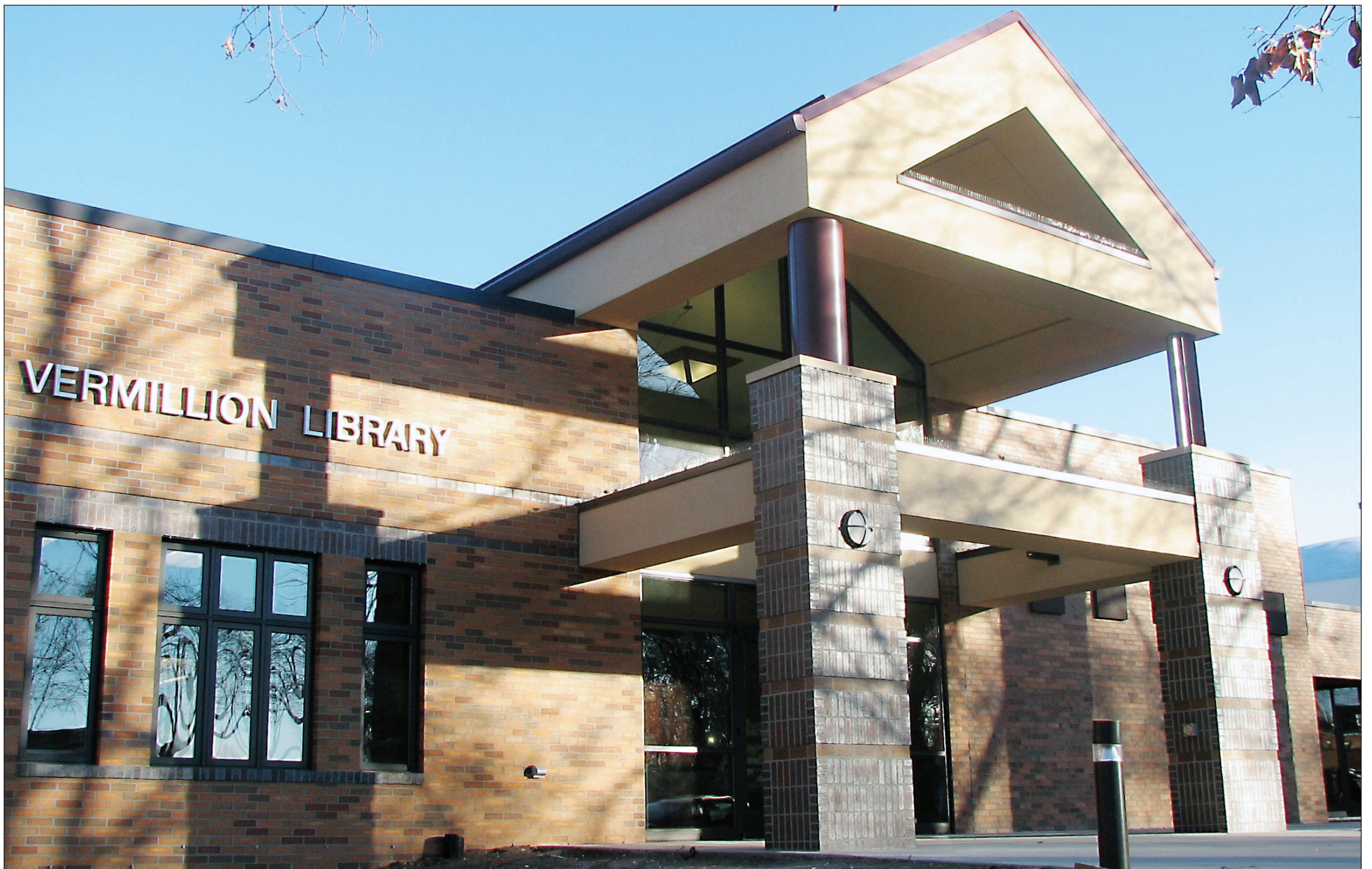
After a two-week moving period, the Vermillion Public Library re-opened Nov. 19, giving patrons their first glimpse into the newly-construct portion of the building.
