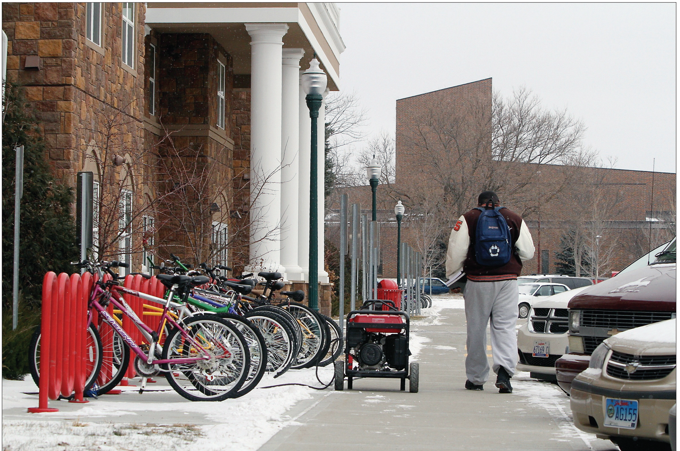
A student walks past a small generator operating outside of Coyote Village near the building's south doors Tuesday afternoon. Students were able to return to their rooms during the day long enough to retrieve needed items.
