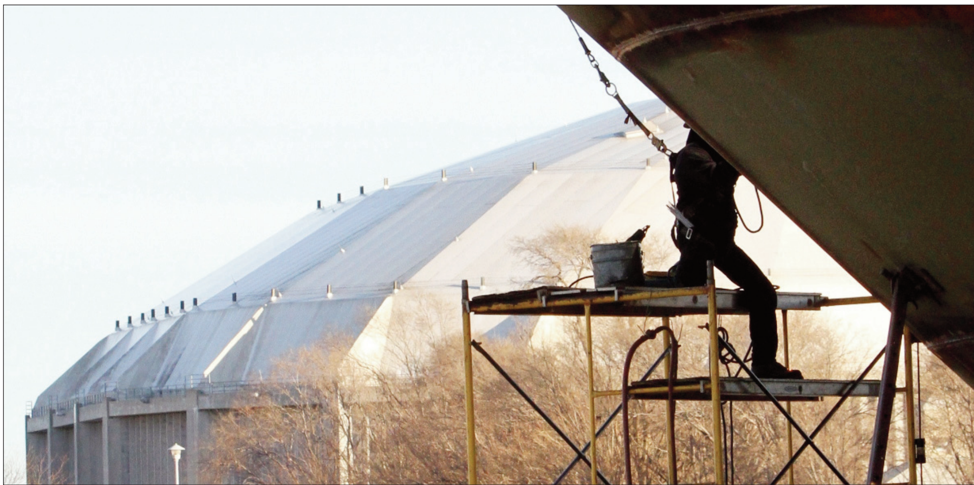
A welder from Maguire Iron, Inc. of Sioux Falls works on the bottom of the bowl of the city's new water tower Friday, Dec. 27, before it was raised by a crane high above the ground. The welders worked in pleasant 55-degree weather on Friday, but had to cope with high winds and sub-zero temps and windchills that moved in the following day.
