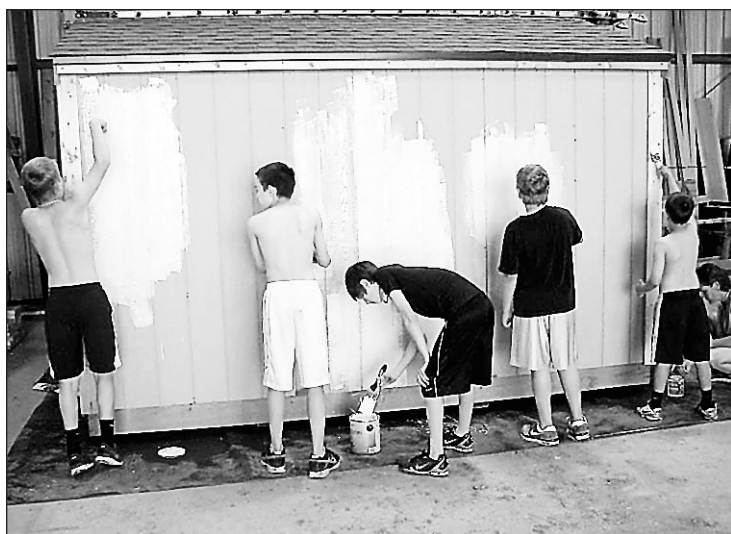
Last month, members of the Vermillion Youth Baseball Association's U12 Travel Team painted a shed to be placed adjacent to a new batting cage near Barstow Park in Vermillion. Herren-Schempp Building Supply donated the paint and the majority of the shed, as well as the use of their storage area in which to paint the shed. Other donations were received from Masaba, Coca-Cola, Jones' Food Center and Ace Hardware. The Vermillion Youth Baseball Association serves 150 Vermillion-area youths.
