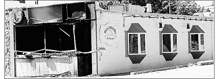
A fire that heavily damaged Recuerdo's Mexican Restaurante in downtown Vermillion is currently being investigated by the South Dakota Fire Marshal and local law enforcement.
