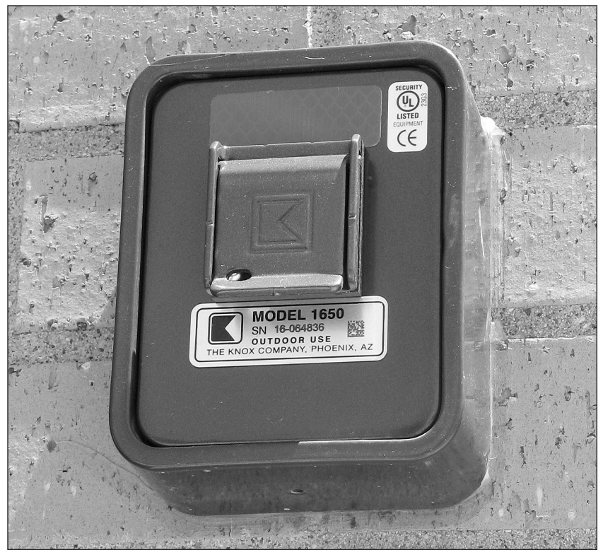
The Vermillion City Council has approved an ordinance that will require a Knox Box to be installed on certain new buildings. The box pictured here is located near the entrance of City Hall.
