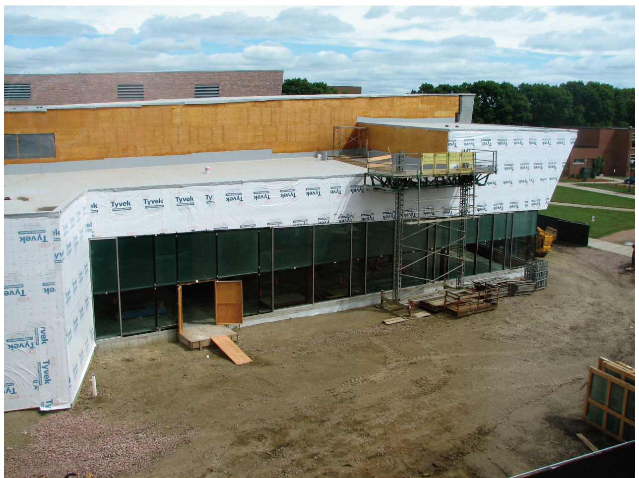
The 31,000 square foot expansion of the Muenster University Center (MUC) began late last fall, with exterior work. Through the spring and summer the project has included placement of additional steel beams, pouring the floors, and work on the exterior enclosure of the new addition. (Photo by Travis Gulbrandson)
