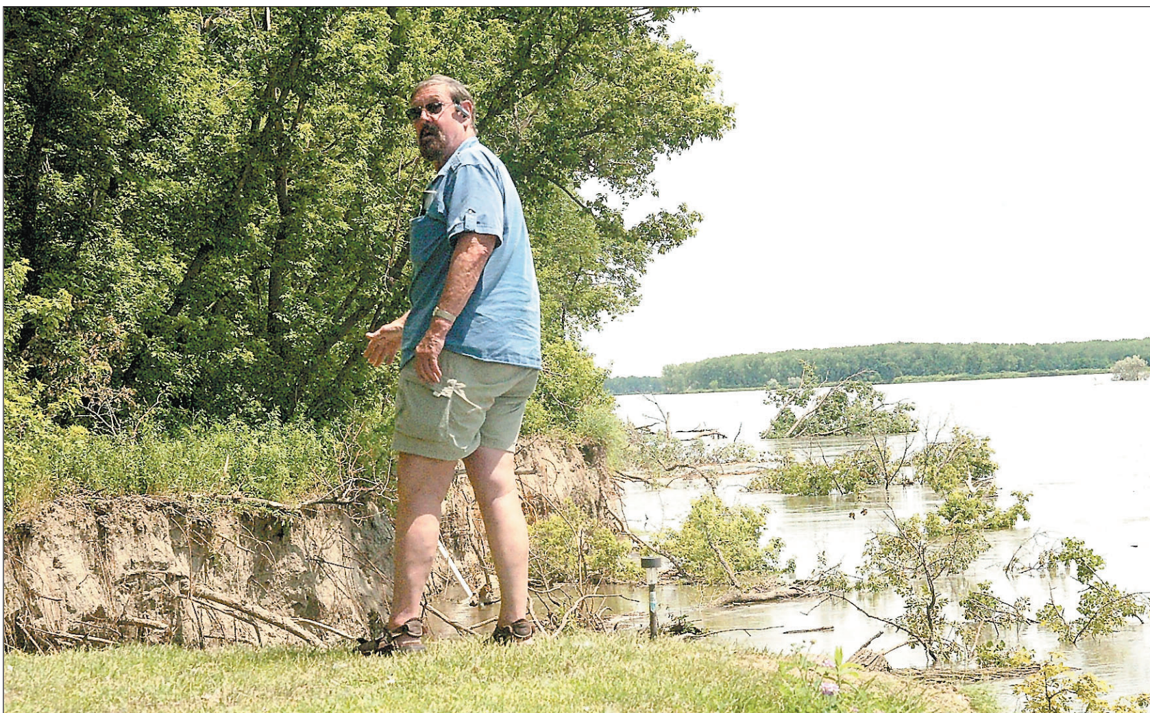
Larry Brady observes the havoc that a high, fast-flowing Missouri River can wreak. This stretch of bank near the Ponderosa housing development, seemingly stable with a thick growth of trees, was stripped away by the churning water in 30 minutes time. Homeowners took action to stabilize the bank near their properties so they wouldn't also succumb to the river.
