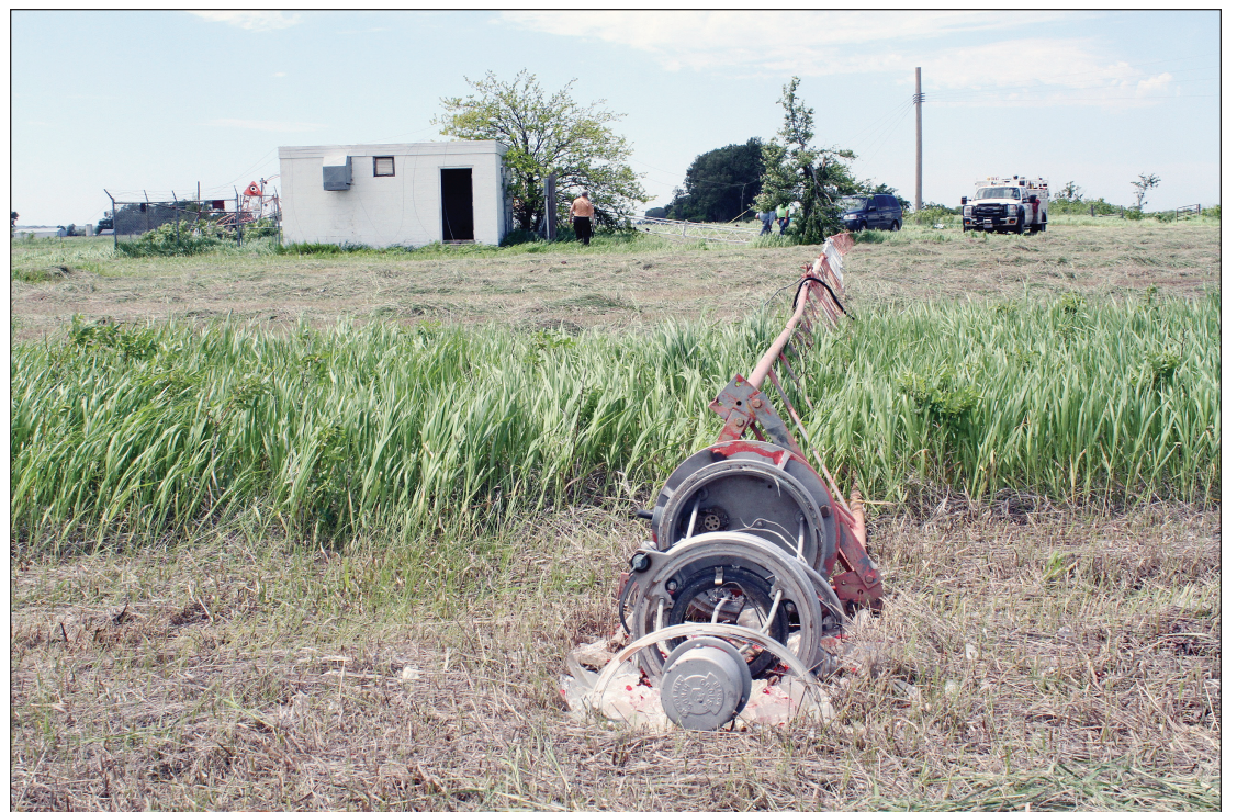
Engineers scrambled Tuesday to find the best way solution to getting KVTK-AM's radio signal broadcasting again after the station's tower collapsed Monday.
