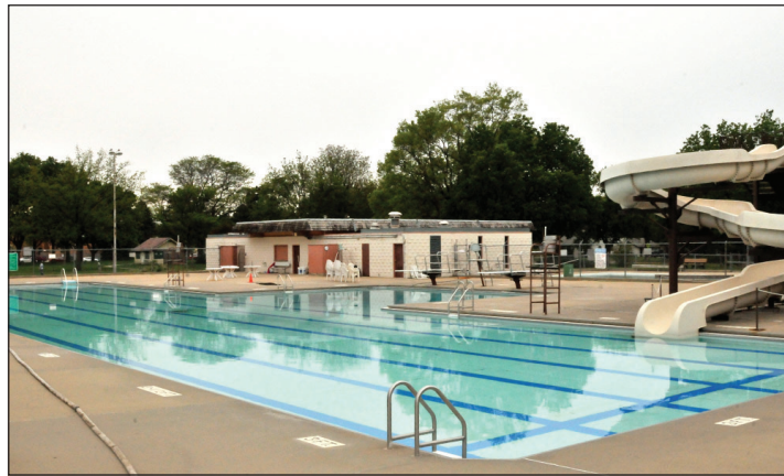
SHAUNA MARLETTE/FOR THE PLAIN TALK Prentis Park Pool is ready to open for the summer Saturday at 1 p.m. (weather permitting.) It is then scheduled to close on July 31 in order for demolition to begin for the new swimming pool scheduled to open the summer of 2016. However, the vote scheduled for June 30 could have ramifications on just what will be built during the next year.
