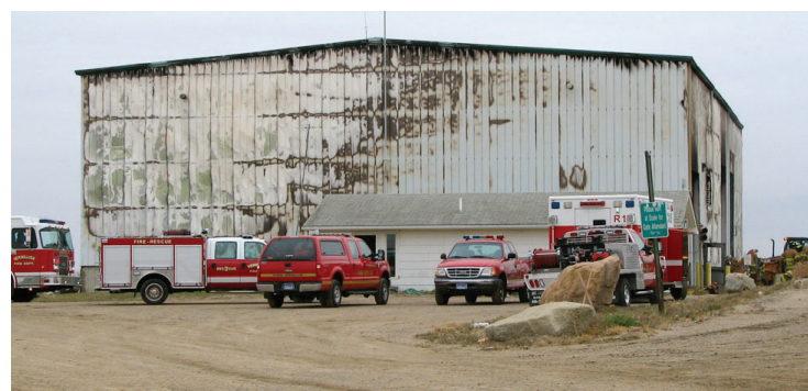
The baler building at the Vermillion Landfill stands charred after an early-morning fire Oct. 22. The cause of the fire is undetermined. (Photo by Travis Gulbrandson)
