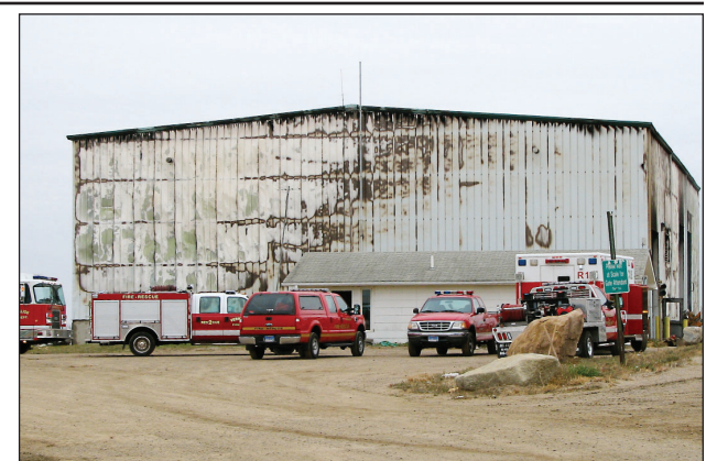
The baler building at the Vermillion Landfill stands charred after an early-morning fire Monday. Four fire departments cooperated in extinguishing the blaze.
